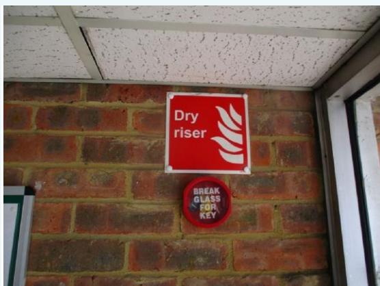
*Signage indicating the location of the dry riser inlet is clearly visible. The cupboard was locked and a key is available within the entrance of the property.*
