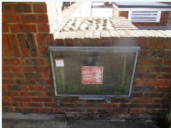
*A dry riser is installed, with an inlet at the front of the building and outlets on each floor.*
