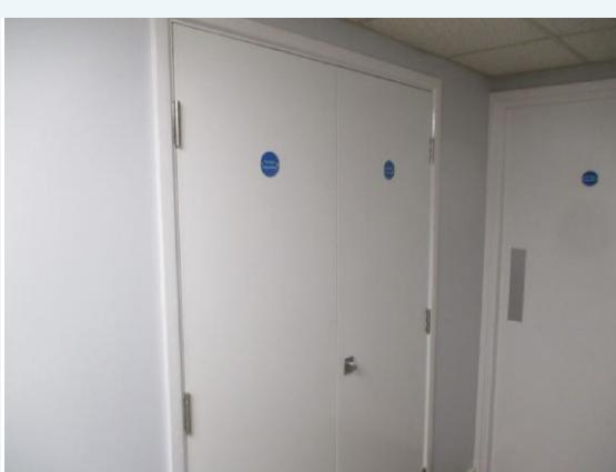
*Electrical distribution is enclosed within a suitably fire rated cupboard.*
